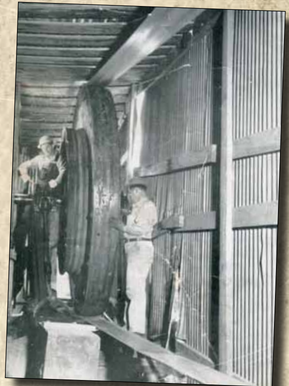
Roustabout A. J. Yost and gang pusher A. I. Abercrombie tighten up jack post on vertical band wheel at Sutton A-5 well, Fairpoint, Kansas. This giant old-style wooden wheel, reminiscent of earlier days in the oil fields, is no longer common, more modern pumping equipment have superceded it in most of the newer production areas. (Photo from the July, 1945 SOHIOAN magazine.)
